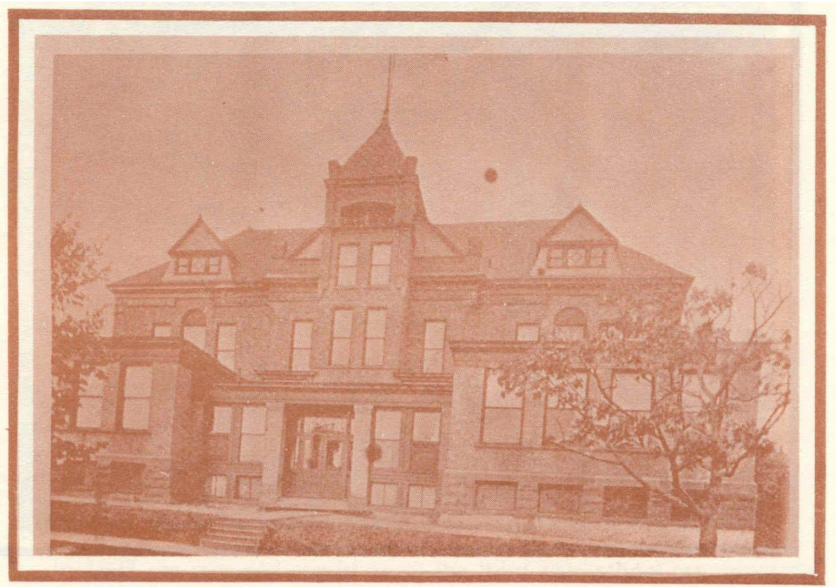
Old Washington Elementary School
